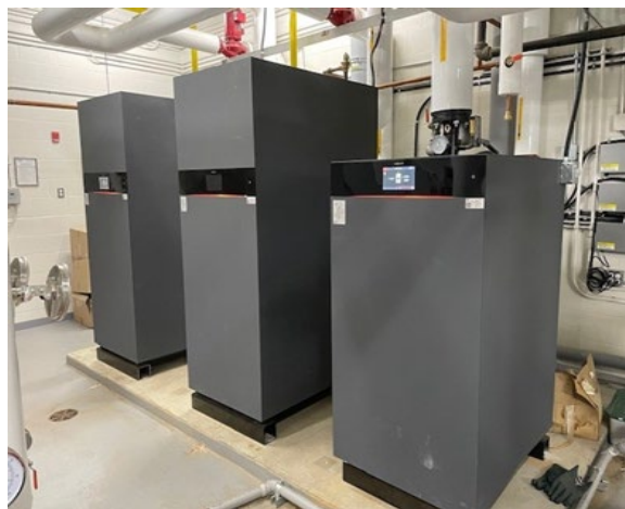
CPAC boiler replacement
