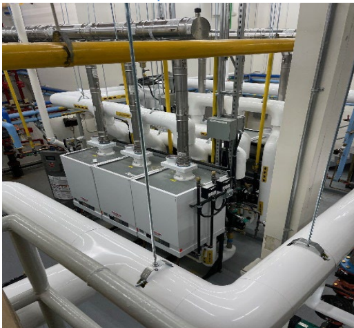
Riverside boiler replacement
