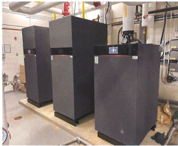
CPAC boiler replacement
