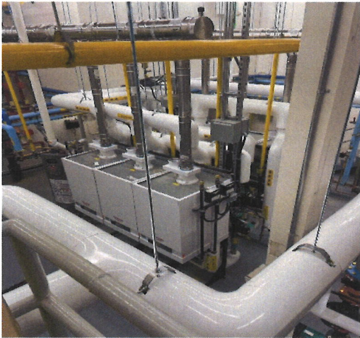
Riverside boiler replacement
