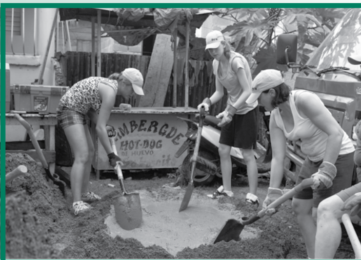
Students mixing concrete
