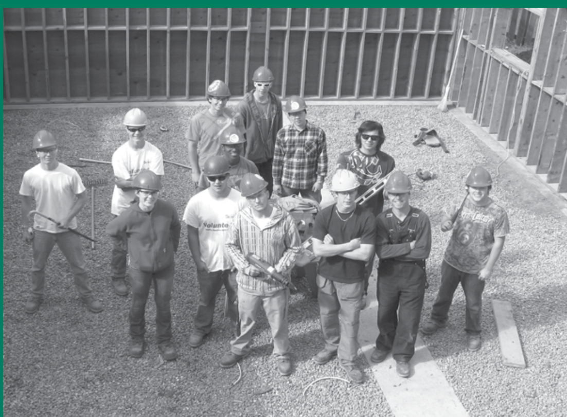
CCAP Students begin foundational work.
